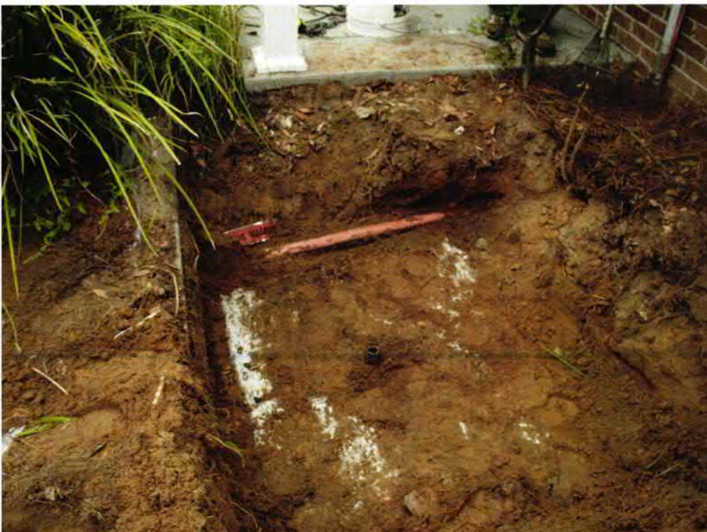
Picture 2: UST 337Ash excavation in progress.
